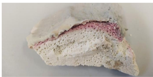
Figure 1. Appearance of the JM26 wall refractory operating at 1185°C for 5 years.
